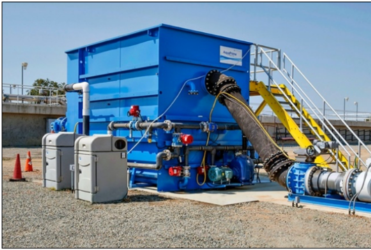
Figure 2. Primary filtration system at the Linda Wastewater Resource Recovery Facility in Olivehurst, Calif. Left photo shows the cloth disk primary filter tank and the photo at right shows the eight individual cloth disks in the filter tank, with a chain drive used to rotate filters during a backwash cycle.
